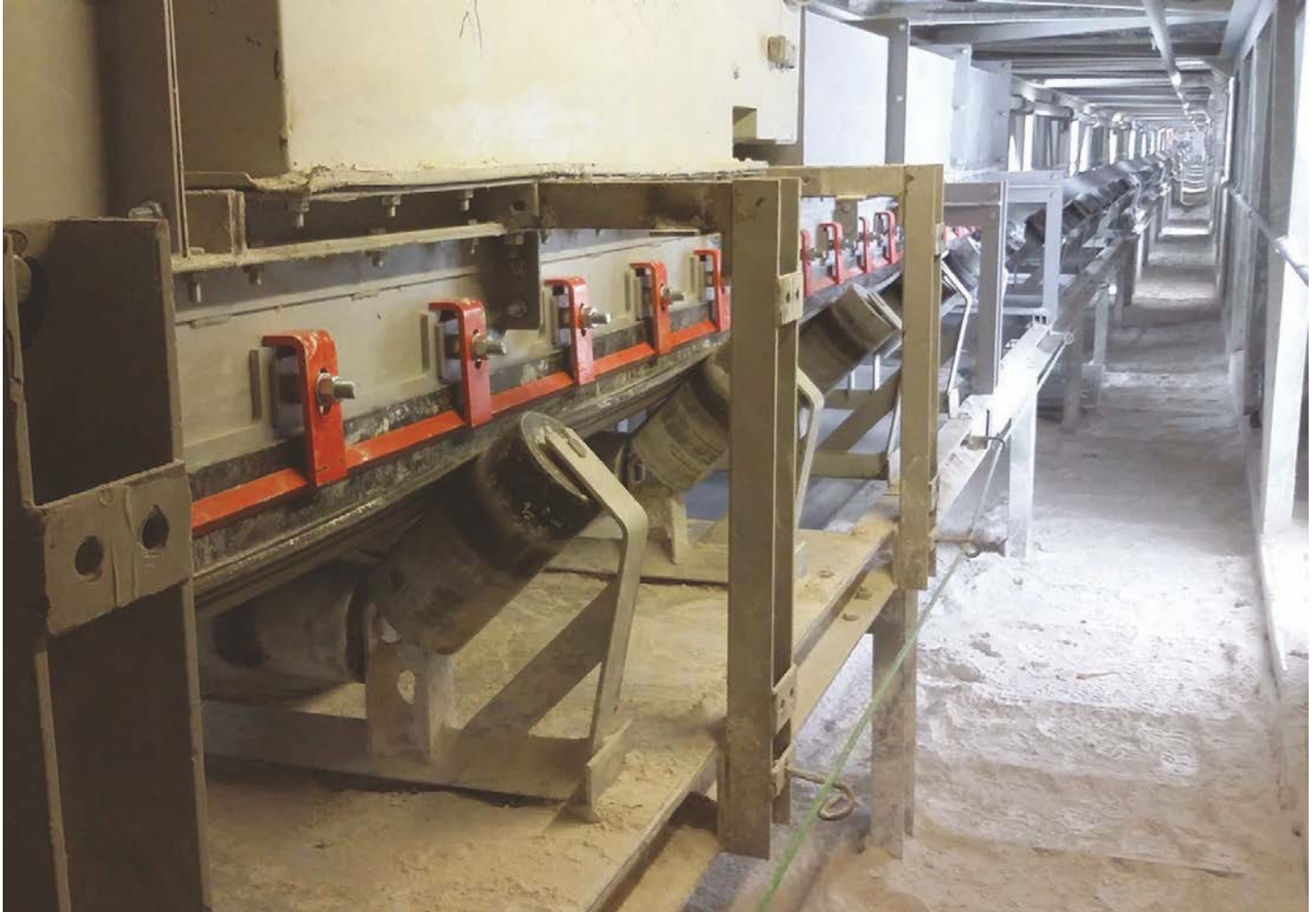
Skirt sealing contains small lumps and fines. ▲
